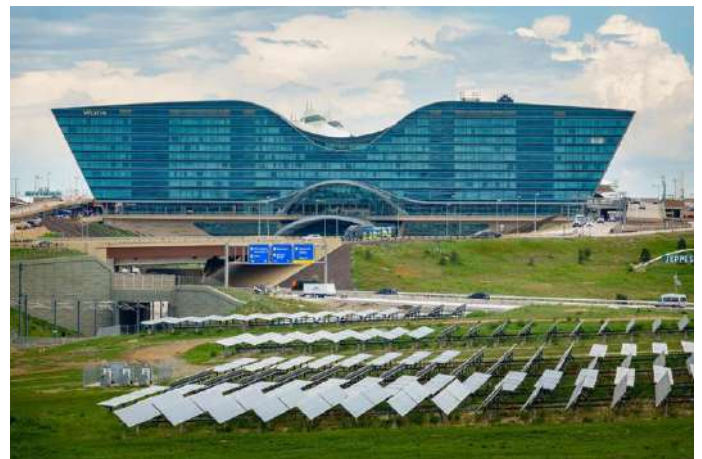
Fig.1: Solar photovoltaic system installed at Denver International Airport.
