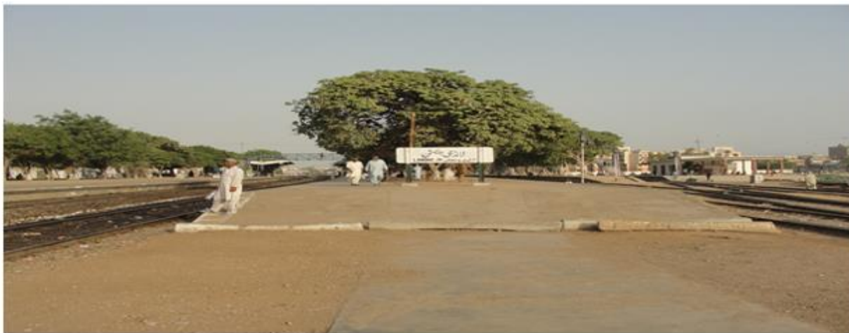
Fig.5. Landhi Junction Railway Station.
