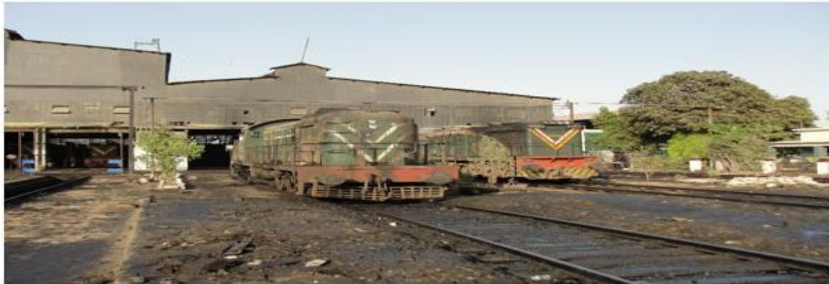
Fig.2. Railway locomotive diesel engine workshop at Karachi Cantonment Railway Station.
