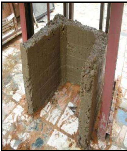
Plate (8) Precasted concrete canal-let
