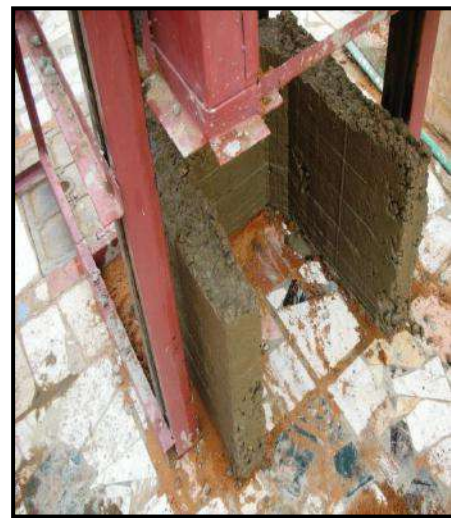
Plate (7) Removing out of inner form
